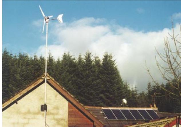
This is a typical kind of arrangement: Small wind power and PV go together very well, *because the wind often blows when the Sun doesn't shine very much*. This shows how different kinds of renewable energy technology can complement each other.
