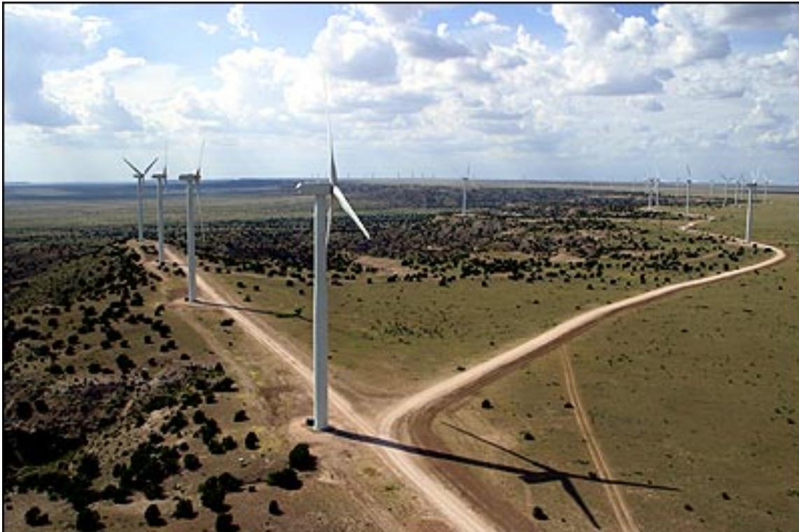
**Utility-scale Wind Turbines are Incredibly Large and Powerful:** A utility scale wind turbine is an amazing machine. Typical turbines are over 200 feet tall, and have rotor blades longer than 100 feet (see photo below). A utility-scale wind turbine is like “a 747 on a stick!”
